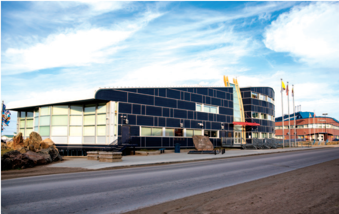
Designated Building 926, the Legislative Assembly of Nunavut building serves as the seat of the Legislative Assembly of Nunavut.
